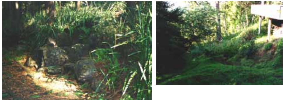
Figure 10 (left): View of the Formal Garden spring that drains through the grotto and into the rectangular pool.
